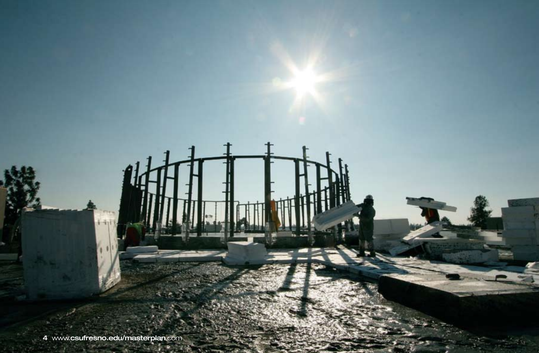
What resembles a modern Stonehenge in this rooftop view of the expanded Henry Madden Library is the structural steel that will form the signature tower.
